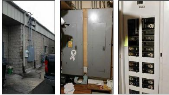
EXISTING SERVICE PHOTOS - SWEDISH INN FAMILY RESTAURANT
