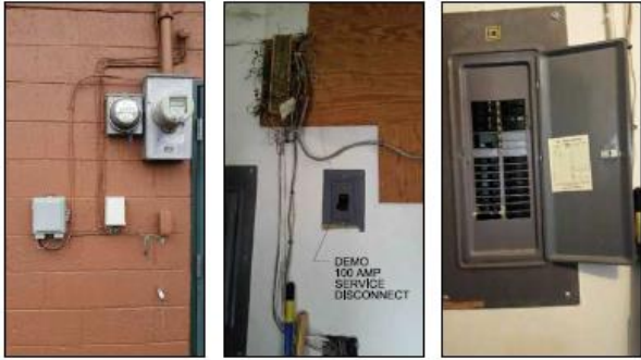
EXISTING SERVICE PHOTOS - VIRGA CHIROPRACTORS
