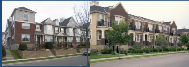
Multi-family residential should include features such as individual entrances, porches, and gables
