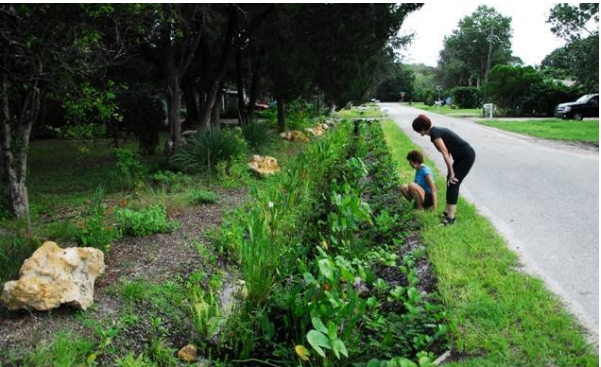
Bioswale Along Roadway
