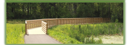
Allemansrätt Park Bridge & Boardwalk Projects
