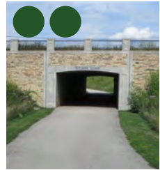
TRAIL THROUGH BOX CULVERT
